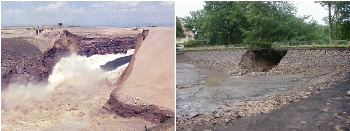
Fig. 1. (a): The catastrophic failure of the Teton dam (U.S., 1976); (b): The breach of the Ouches dam (France, 2001)
